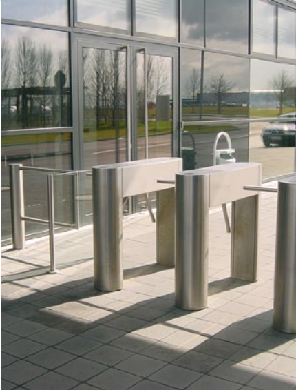
Access to company site, outdoor installation
